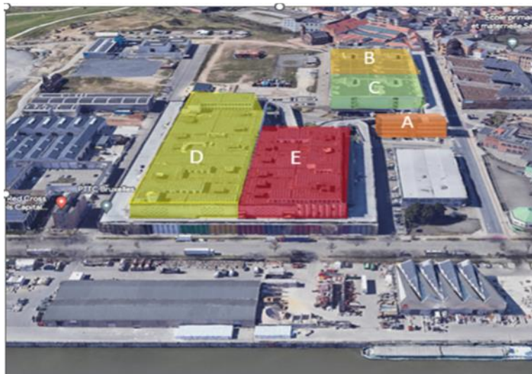
TIR site with the various buildings (A, B, C, D and E)
